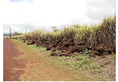
7.7.12 Right perimeter of easement overgrown
